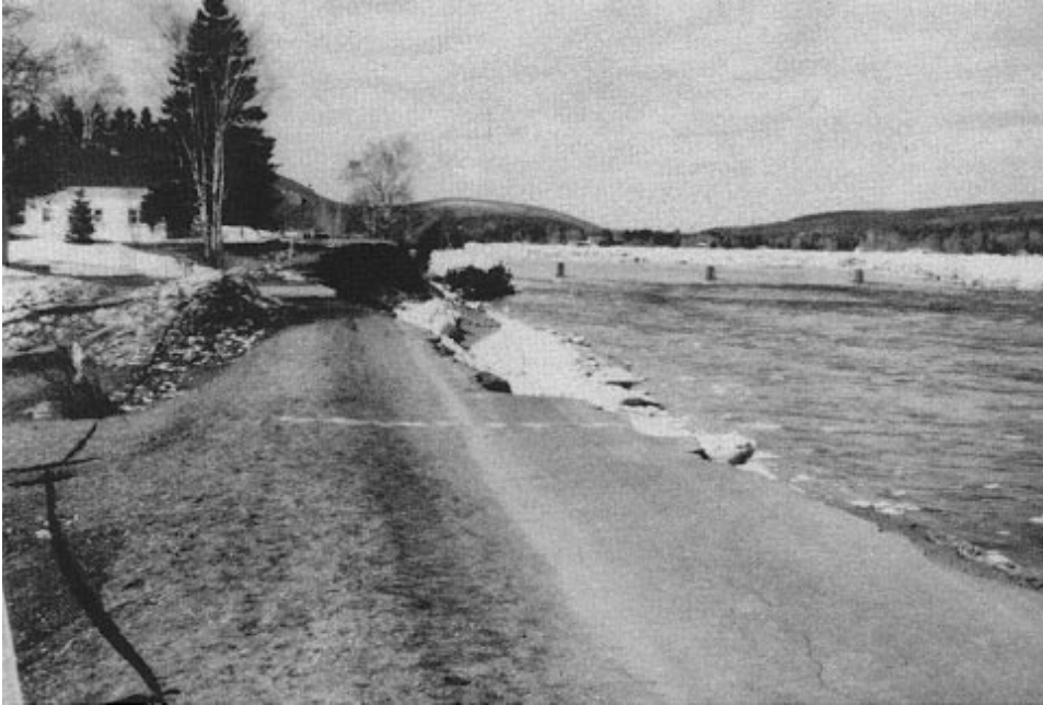
Figure 2-6. Bank scour due to a breakup jam, St. John River, MN, near Allagash
